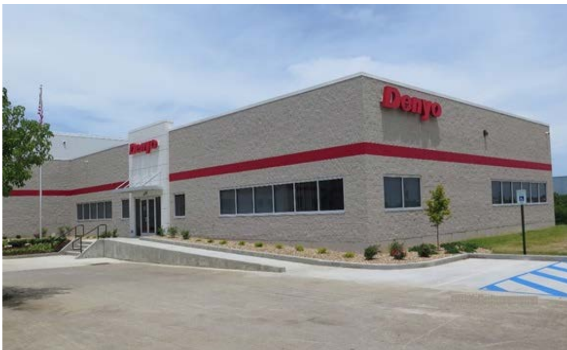
写真 : Denyo Manufacturing Corporation (U.S.A.)
