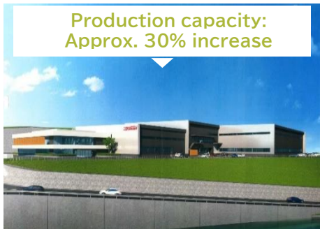
New head office plant of Nishihatsu Co., Ltd.
