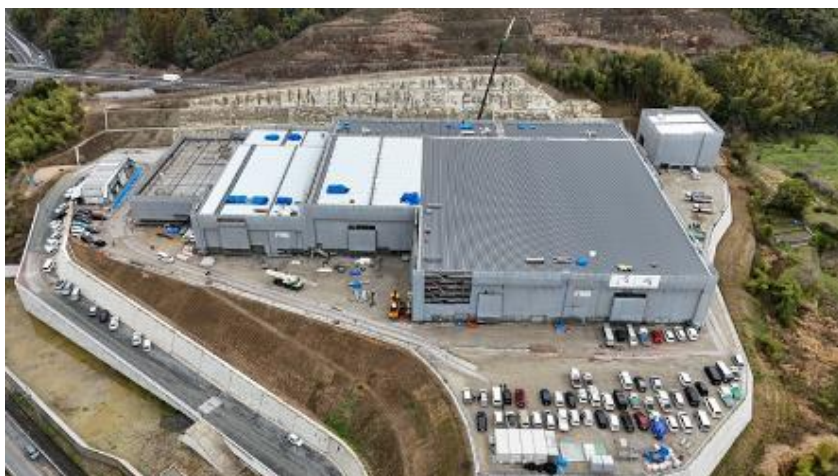
Completion of Nishihatsu's new head office plant is scheduled in FY2024.
