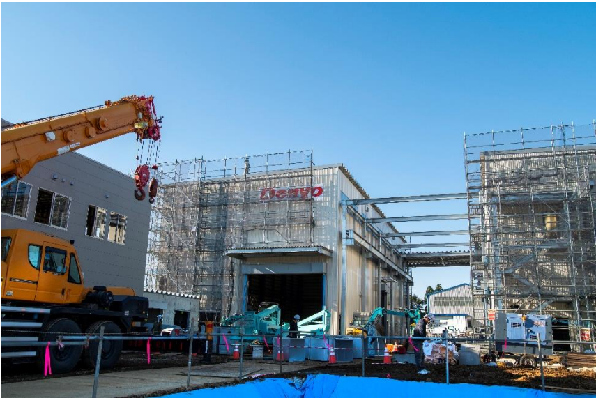
Large repair base under construction(Sakura City, Chiba Prefecture)
