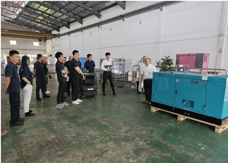
Operation of an installed power generator(Singapore)
