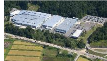
Fukui Plant of Denyo Co., Ltd.
