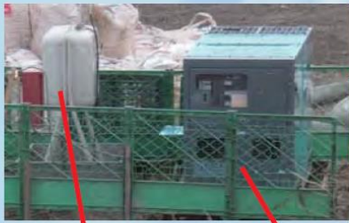
Extend fuel tank Generator
